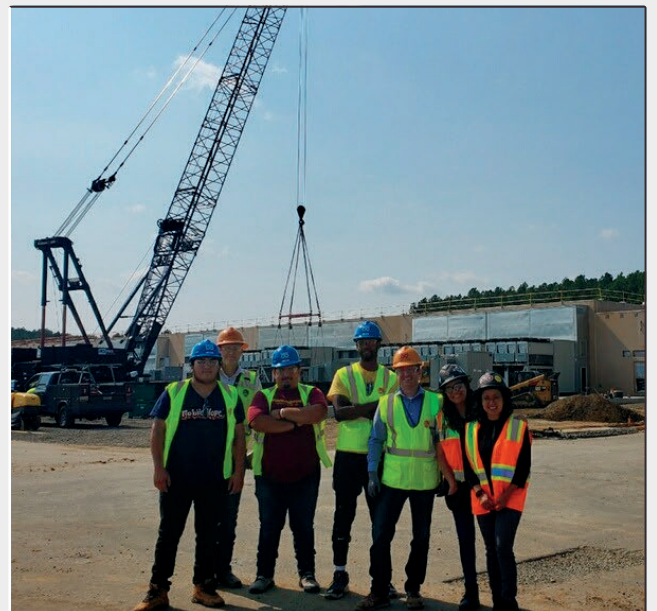
Trade school students visit a construction site to learn about multiple trades.
